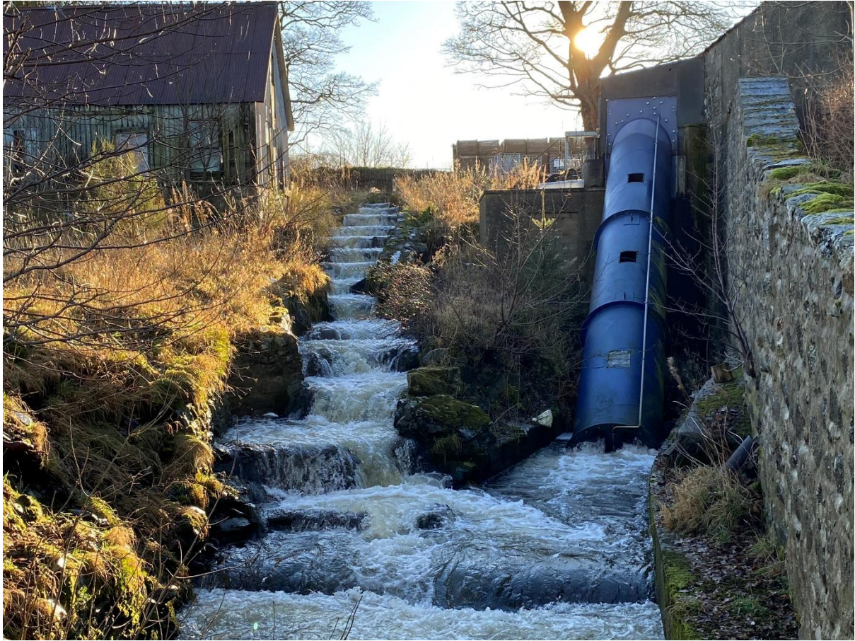
Figure 7. Lady Anna Falls step pool fish pass on left and hydro on right.
