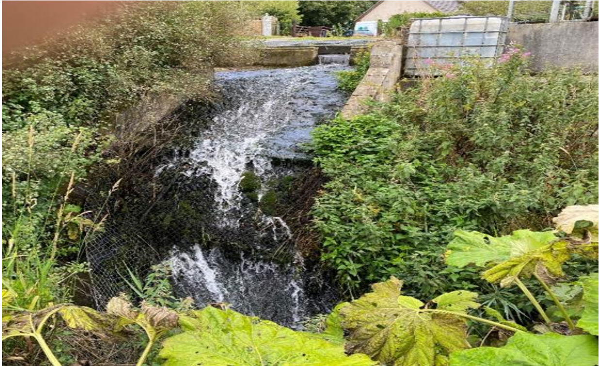
Fig 4, Spillway from hydro scheme.
