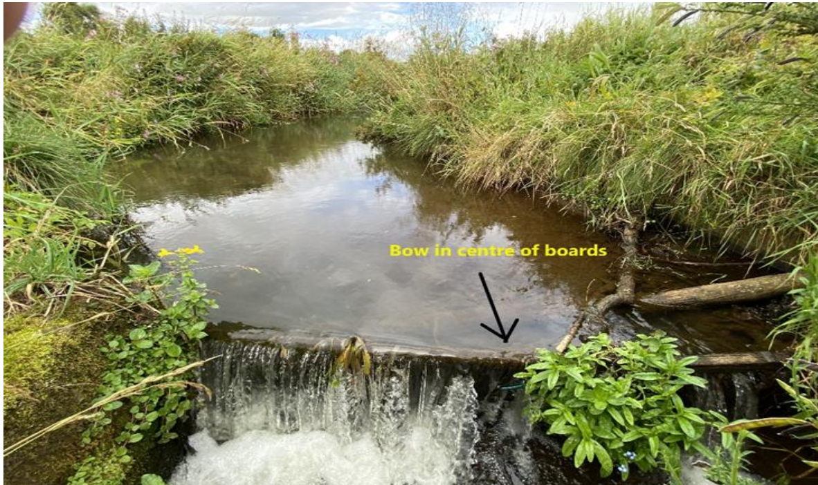
Fig 2, above showing bow in centre of boards at top of abstraction channel
