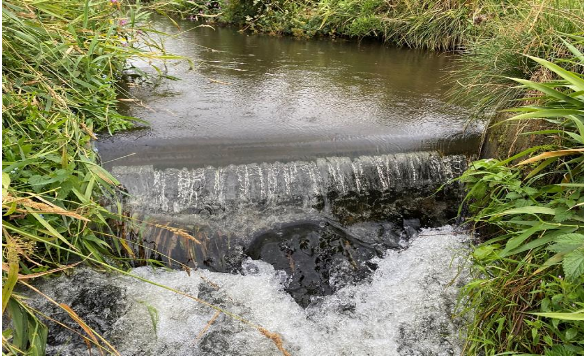
Fig 3. Below showing boards placed at the top of the Ebrie burn channel causing obstruction.
