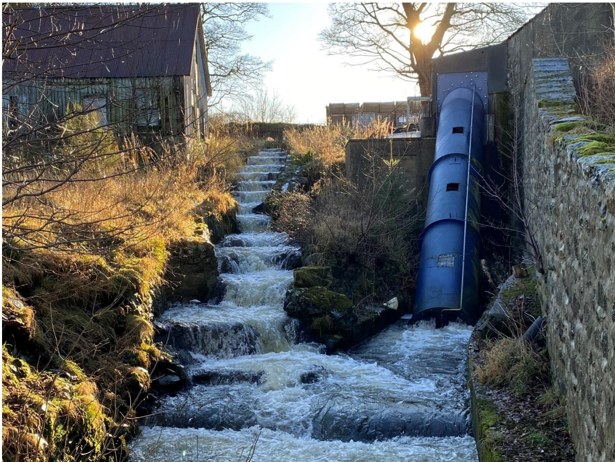
Hydro scheme and step-pool fish pass on the Keithfield Burn
