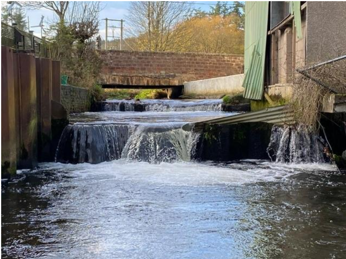
Figure 6. Two-stage sheet piling weir on the lower Fourdon burn by the village of Fyvie, owned by Scottish Water.
