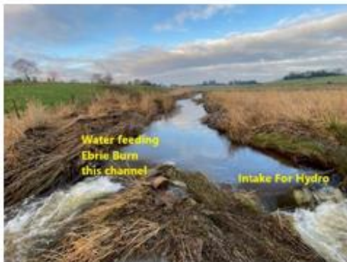
Fig 2, upstream view of Hydro intake.
