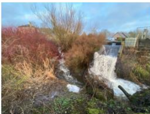
Fig 6, Water Exiting Hydro lade over slip way.
