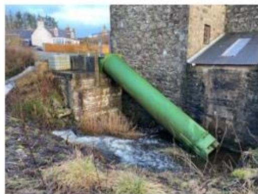
Fig 7, Archimedeian screw not in use.
