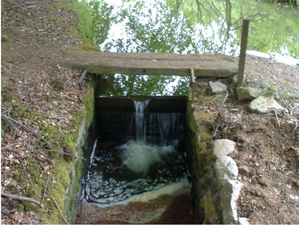
**Keithfield Burn Top Weir. 2012. Shows the sluice. Insufficient Water Going Down the Channel.**
