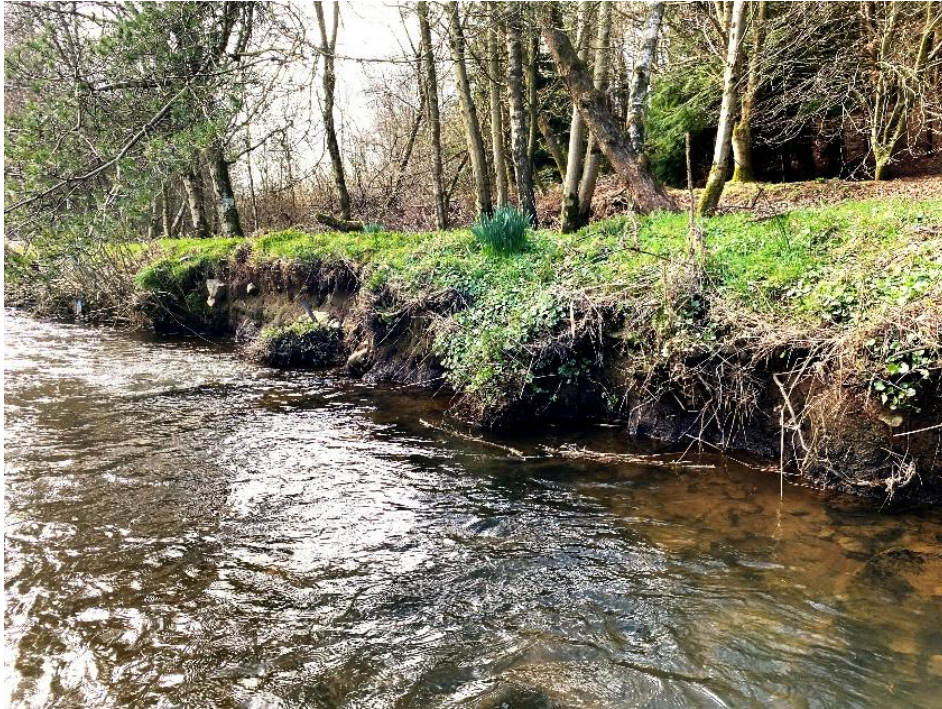
Fig 1, Before repair, very badly eroded bank. 3ft of embankment gone.
