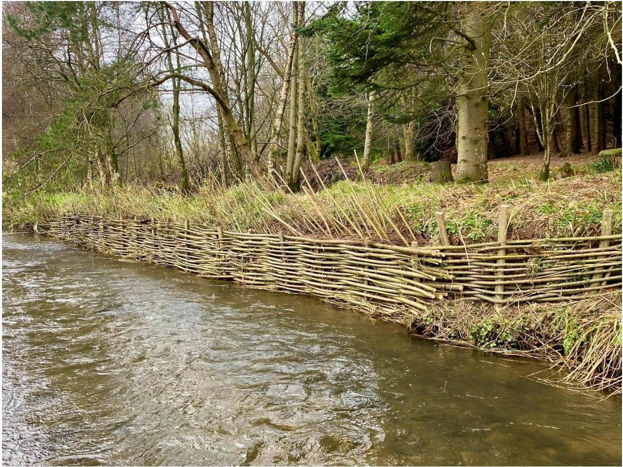
Fig 3, Willow bank repair completed.
